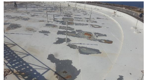
Floated roof initial condition
