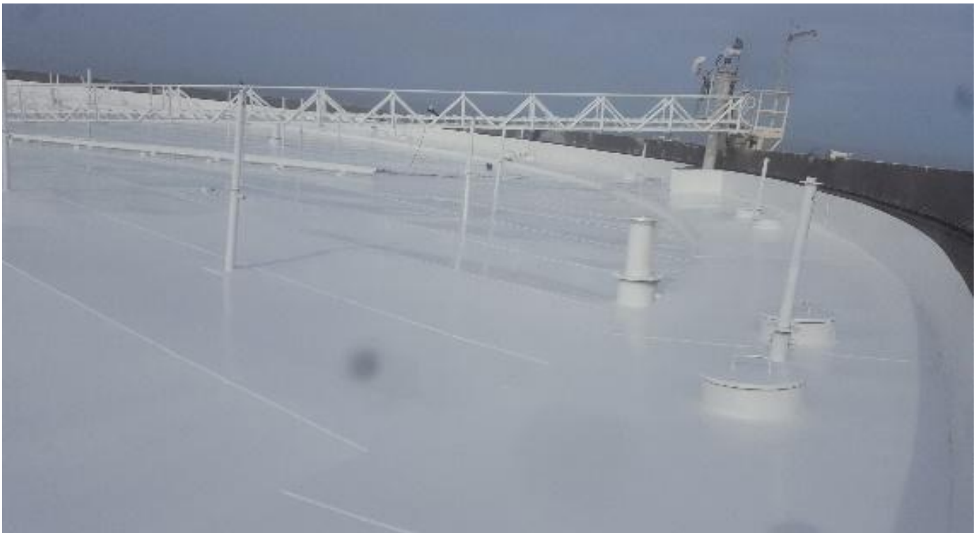
Floated roof appearance after polyurethane top paint
