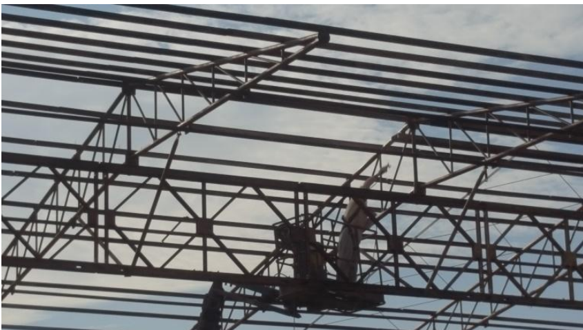
Single layer application with Airless
